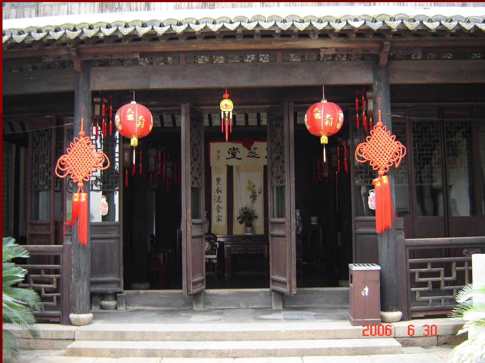
Zhouzhuang – The Zhenbrenjia Hotel: Taken from the middle of the inner courtyard. Notice the raised threshold to keep out spirits and dirt. This used to be a wealthy estate.
