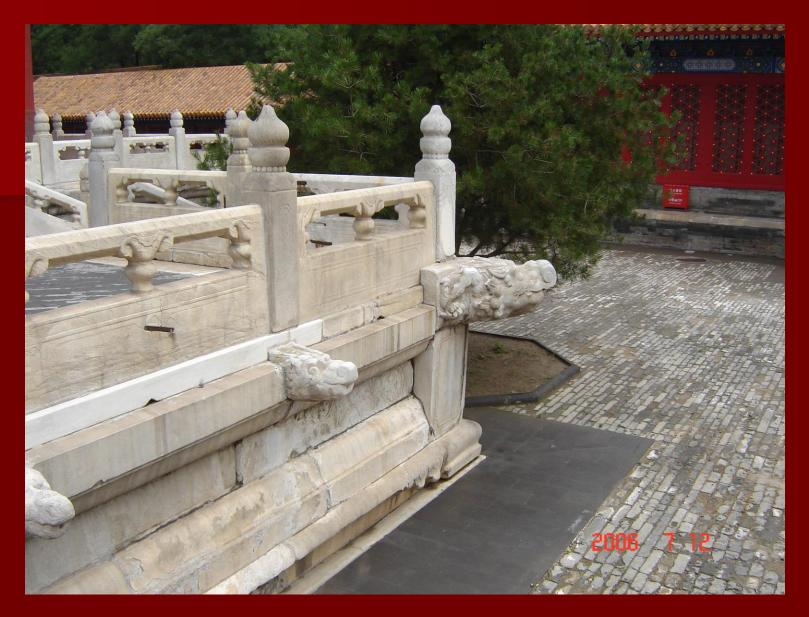
The entire Forbidden City is built on a slight angle so all the rain water drains to the Southeast. These dragon heads act as spouts for the draining water.
