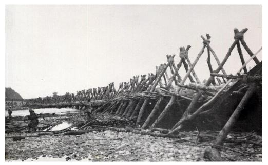
Poles driven into ground provide the frame for the cut-off dam.
