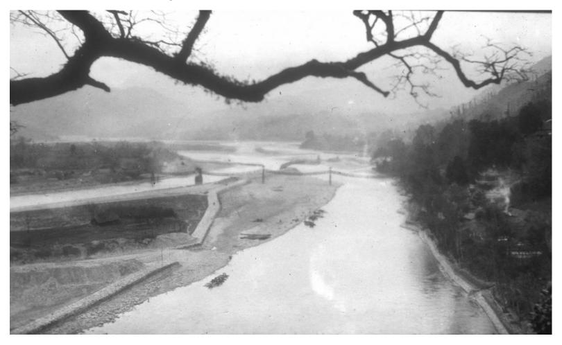
Original canal on left; inner feeder canal on right; "fish snout" or primary division in center beyond suspension bridge; cut off dam blocking inner feeder canal; temple to Great Yu on hillside.
